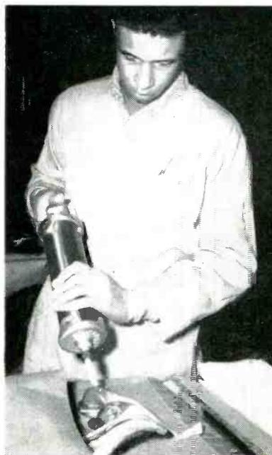
Injecting rubber compound to form plug body around cables and connector
